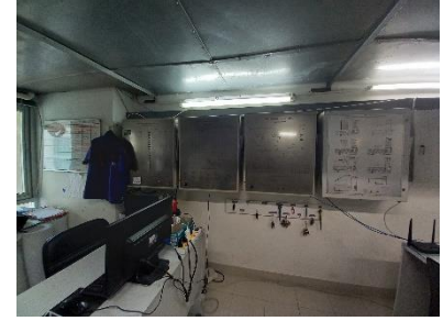
Graphic Annunciator Fire Alarm System
