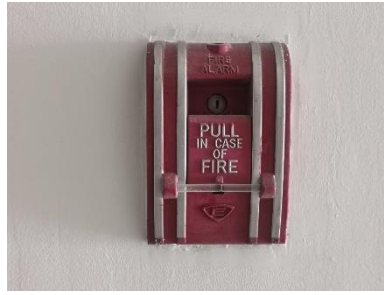
Fire Alarm Manual Station
